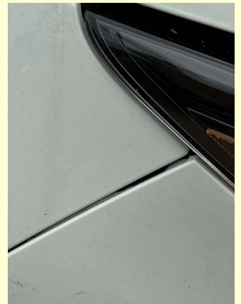
Front bumper cover misaligned
